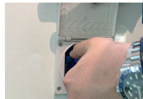
To remove, press the small blue lever with your thumb and pull towards you
